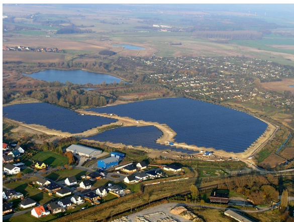
Enerparc 8.6 MW Solarpark in Wismar (2011)
