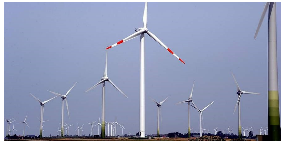
Onshore Windpark Friedrichskoog, 203 MW (2010)
