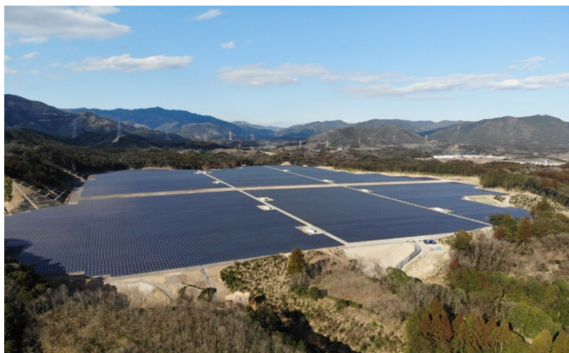
Toshiba 25 MW PV plant in Miyazaki
