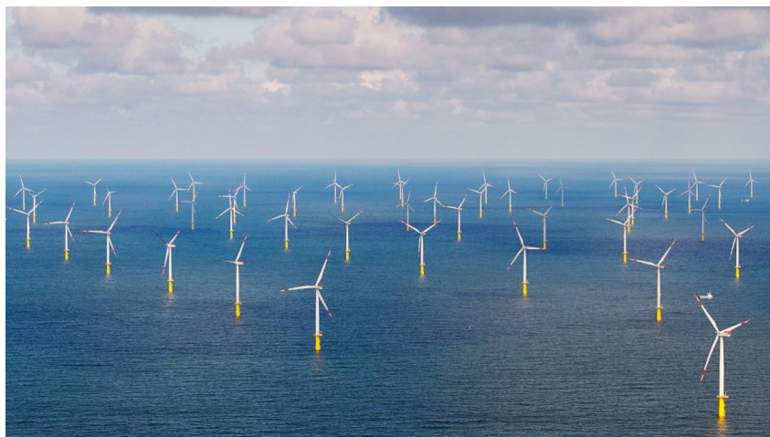
Offshore Windpark Butendiek, North Sea, 288 MW (2015)
